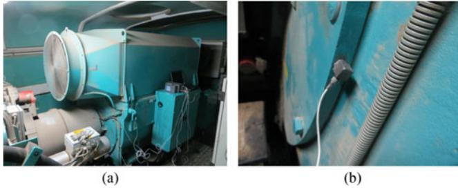
Fig. 19. Generator in the wind field. (a) Overall view of the generator. (b) Position of the sensor.
